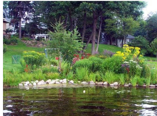
Fig. 8. Sloped artificial erosion control includes rock and riprap, even in minor amounts.
