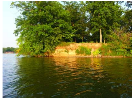
Fig. 4. Severe, localized erosion
