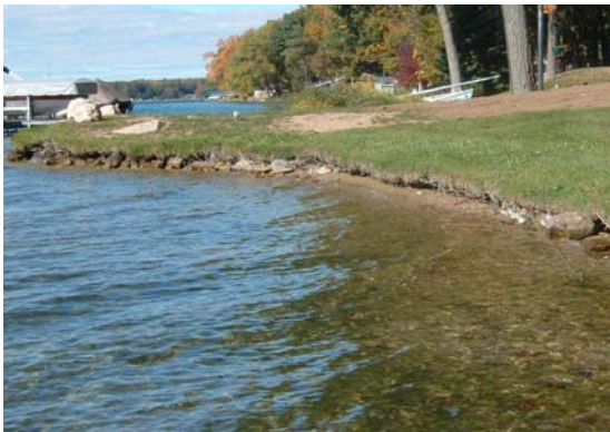
Fig. 3. Moderate erosion, due to extent along quite a bit of shoreline
