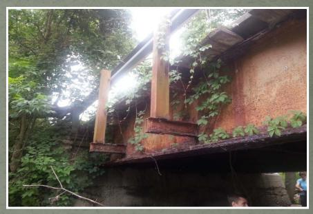
Bridge to be replaced soon Rusted Through Severe Erosion Poor Road Condition
