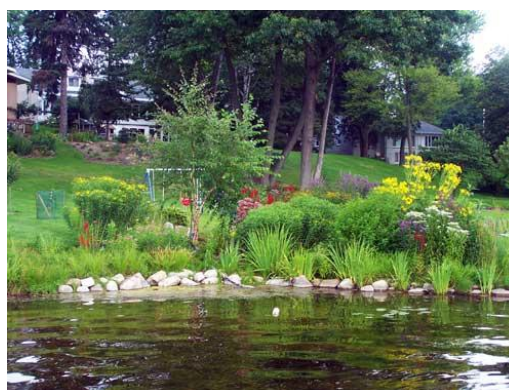
Fig. 8. Sloped artificial erosion control includes rock and riprap, even in minor amounts.
