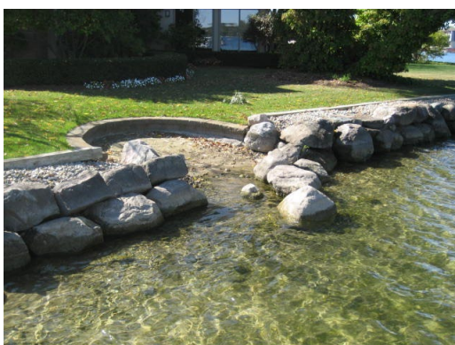
Fig. 7. Vertical artificial erosion control includes seawalls, boulders, and rock walls.
